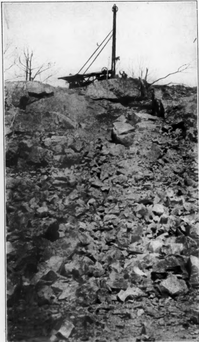
Well Drill at Top of Quarry
